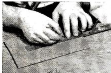
When laying out a panel, base, etc., be sure to make accurate markings by means of a scribe and square
