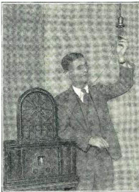
The type of aerial shown here is nothing more than a fixed condenser which is inserted in the light socket.
