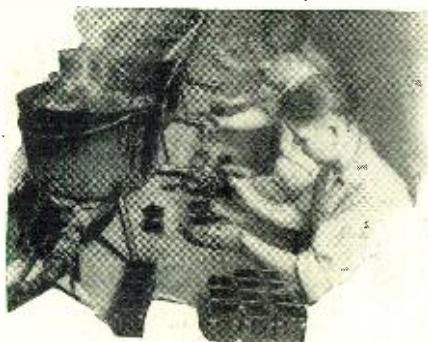
Scene in transformer factory, showing how transformers are filled with a moisture-excluding compound. The compound is kept in a melted state in the big pots, by the gas heaters under the latter, and is simply drained off by means of a spigot.
