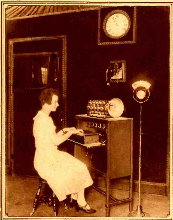
The Pianorad, showing the twenty-five tubes and oscillator circuits.
