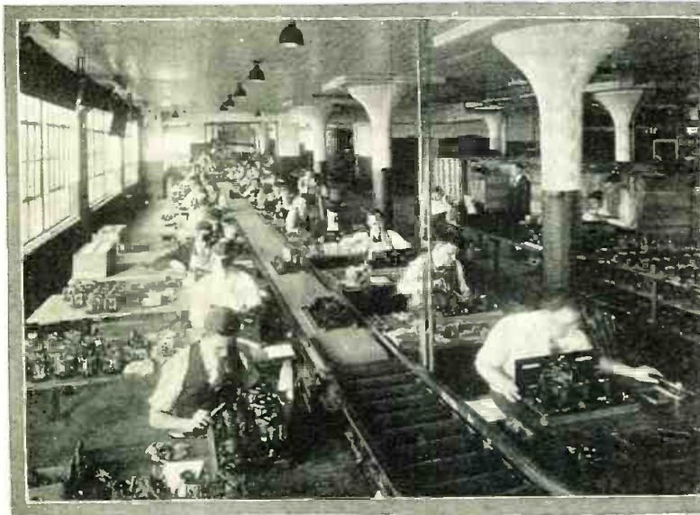
Above is shown the final assembly of the sets, with the operators who wire them. Belt conveyor systems are used throughout the plant; and a section is here shown, carrying the sets from the workers.
