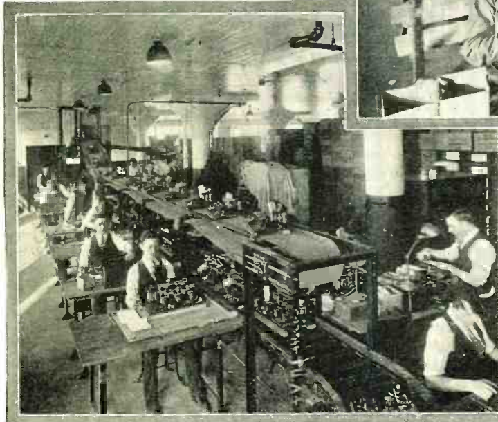
At the right is shown the section of the plant where parts are assembled. In the foreground are operators assembling and inspecting variable condensers.
