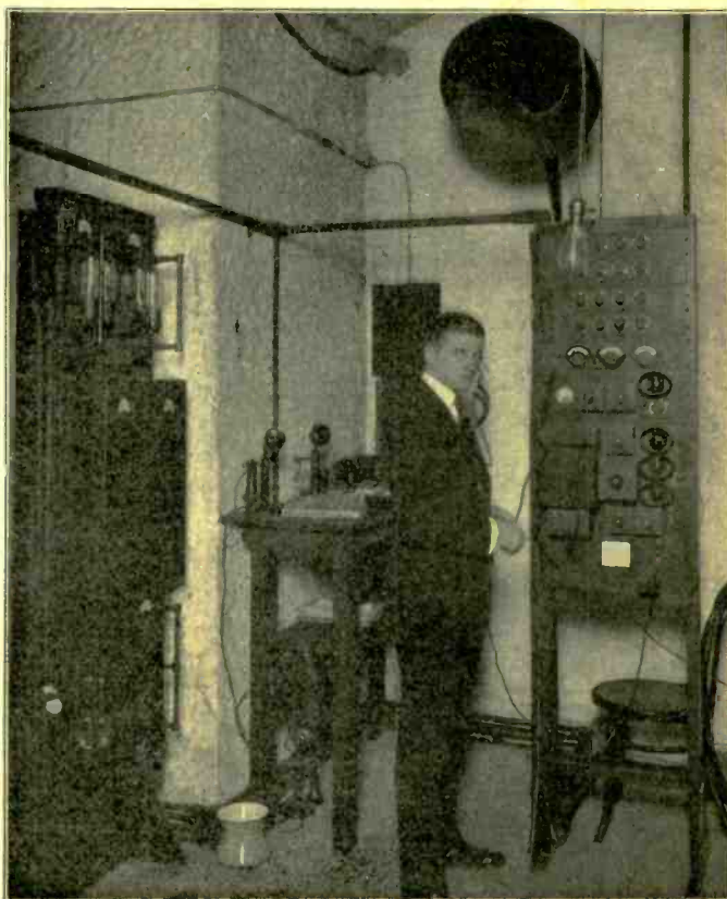
In the Picture Above, Showing President Harding Delivering His Message to Congress, May Be Seen Several Microphones, Outlined with White Circles, Which Were Installed at Various Places to Pick Up the Voice. On the Right is Shown the Amplifying Device Installed in the Cellar of the Capitol by the Western Electric Co. In Front of the Operator is a Speech Amplifier Composed of Four Tubes. The Speech, After Being Amplified by This Apparatus, Passes Into the Second Power Amplifier on the Left Side Panel Upon Which May Be Seen the Four 50-Watt Tubes on Top and at the Bottom, the Last Two Power Tubes of 250 Watts Each. From This Installation, the Voice is Carried Through Wires to the Loudspeakers Installed at Various Places and Also to the Navy Broadcasting Station, NOF.
