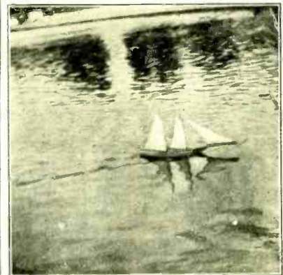
Fig. 17—Echelon Waves on Water Produced by the Motion of a Boy's Model Ship.
