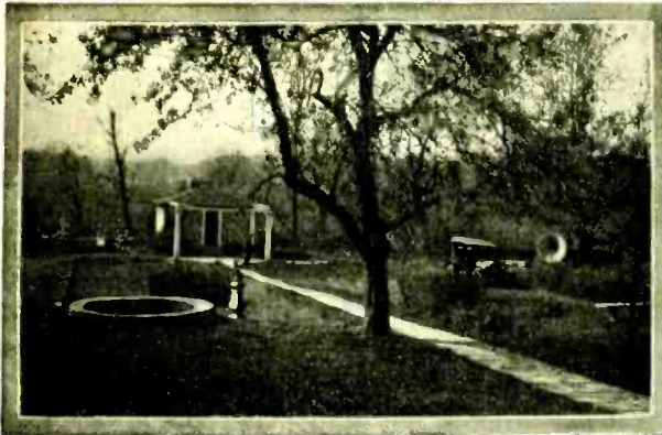
Three Views of the Large Cement and Stone Loudspeaker Built by Mr. M. C. Hopkins of Washington, D. C. The Volume From This Speaker is Sufficient to Carry Sounds Clearly for a Distance of Two Miles. This Horn is 7 Ft. in Diameter.
