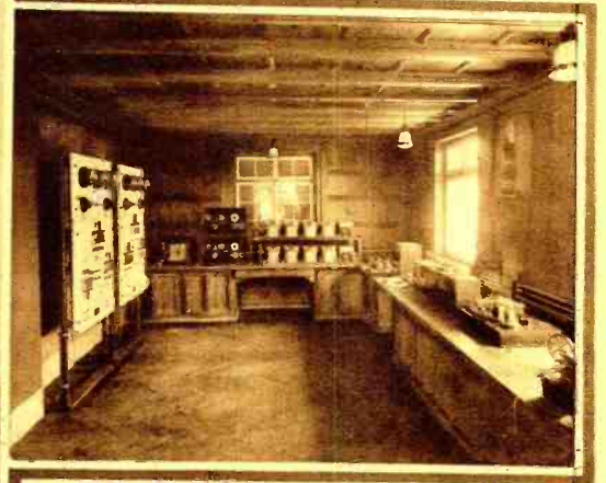
The Central Control Room at the Berne Post Office. Messages Are Received from the Receiving Station Three Miles Away and Transmitted from the Sending Station Six Miles Away. Duplex Operation at 150 Words Per Minute is Conducted.
