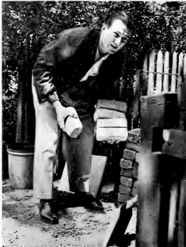
Bricks for a barbecue? Ted's always ready to rebuild anything "nearer to the heart's desire."
