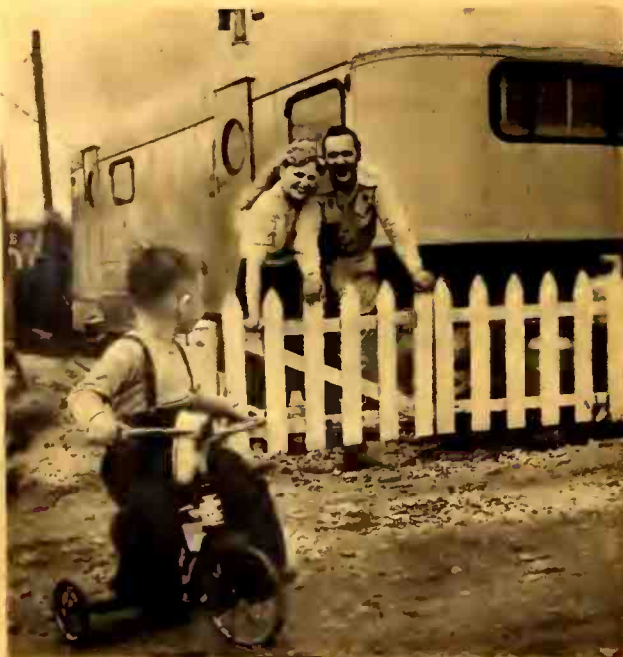
You can easily pick out the Hewitts' trailer on the lot—theirs is the one with the picket fence.
