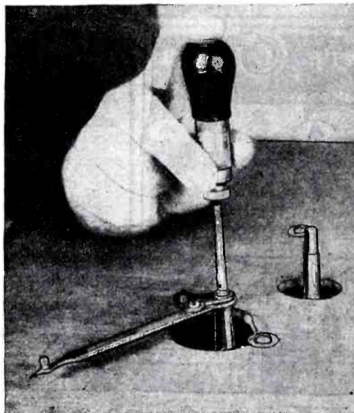
In the photo above, the speed regulator arm of the phonograph motor is being fastened in position on top of the box. The turntable shaft can be seen protruding through at the right.
