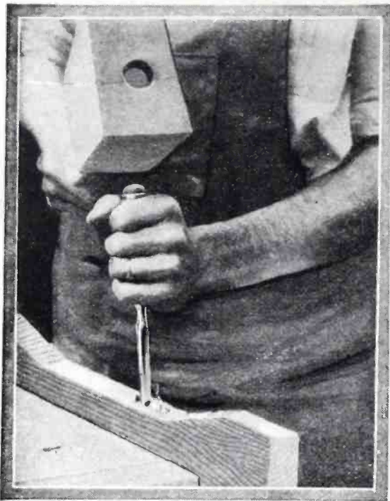
Cutting a mortise.
