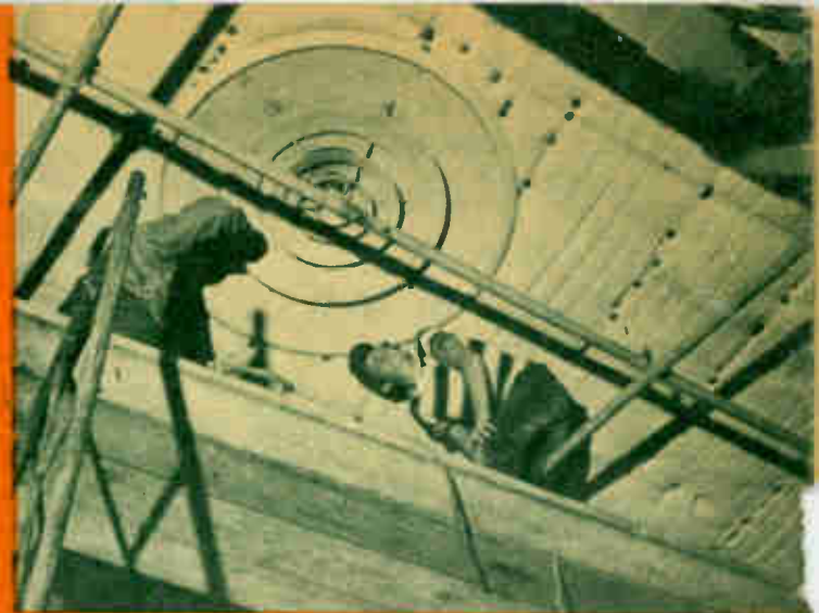
▲ WORKMEN WERE BUSY LAST WEEK installing the large, round "anemostat," a device for spreading cool air throughout a television studio, in NBC's Hollywood television station KNBH (Channel 4). (NBC Ziegler photo.)
