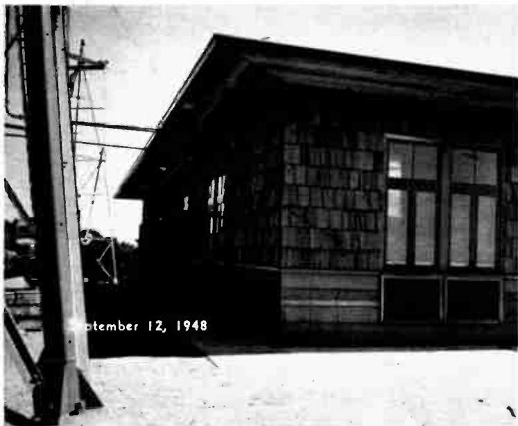
▼ A SHINGLE-SIDED BUILDING WHICH blends artistically into the mountain setting was chosen by KFI for its transmitter operation atop the mountain. Left, foreground, a corner of the towering transmitter. In rear, transmitter of FM station, KVUN, United Garment Workers. Behind KFI-TV transmitter building is two-story structure with accommodations for four staff men.
