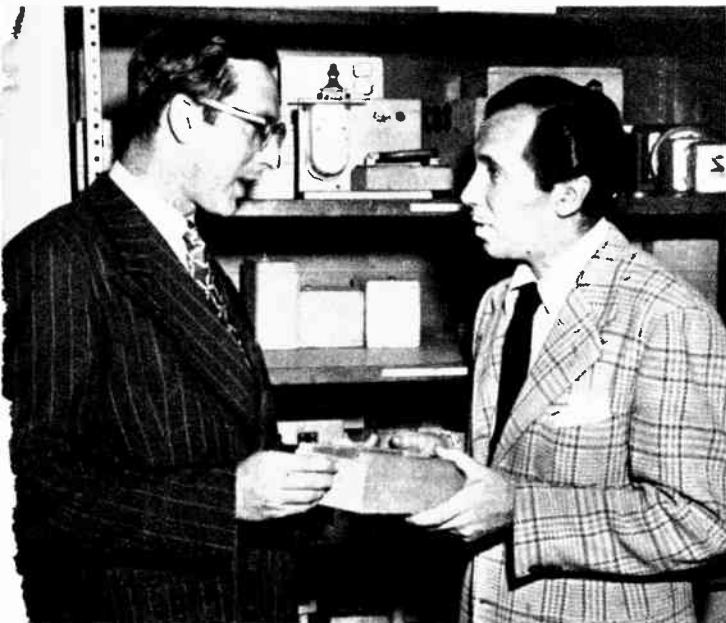
AL SPAN AND SOUNDMAN BERNE SURREY discuss a point concerning one of the hundreds of noise-makers in the department. Al is holding what is called a "bird box." The button on one side of the box makes any one of several bird-calls when it is pressed. Those larks you hear during an idyllic outside scene on a CBS show will come from the throat of a square wooden bird . . . under pressure.
