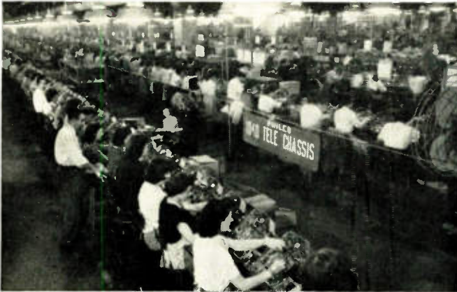
A Philco television assembly line that has helped jump the firm's 1948 production to 360 per cent of last year. Women with nimble fingers are wiring model 1040 TV receiver chassis at the company's Philadelphia plant.
