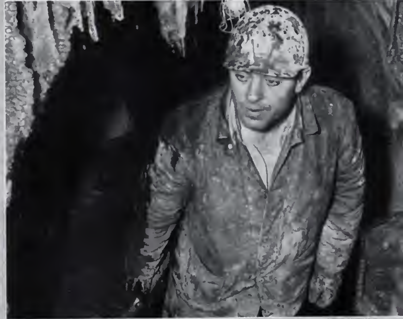
THIS GENTLEMAN and 750 fellow "muckers" digging Chicago's new subway are sandhogs. In N. Y. subway, "Americans at Work" found them working under dangerously high air-pressure, for higher pay as pressure increased
