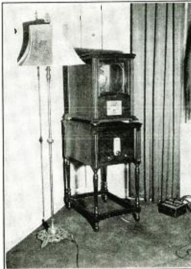
Complete home receiver equipment, DeForest-Jenkins, for sound pictures.
