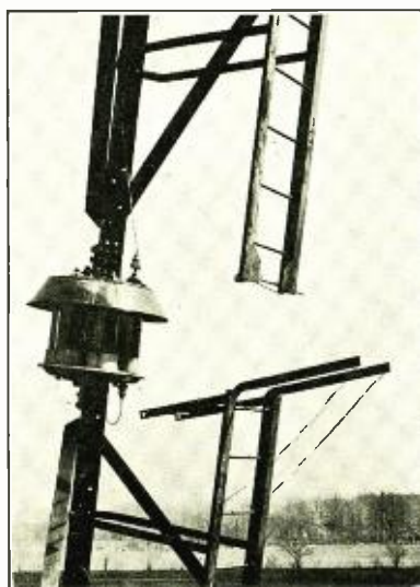
Fig. 1. Detail of ladder and lighting in WHK tower.
