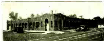
The new Jenkins and Adair plant, in Chicago.
