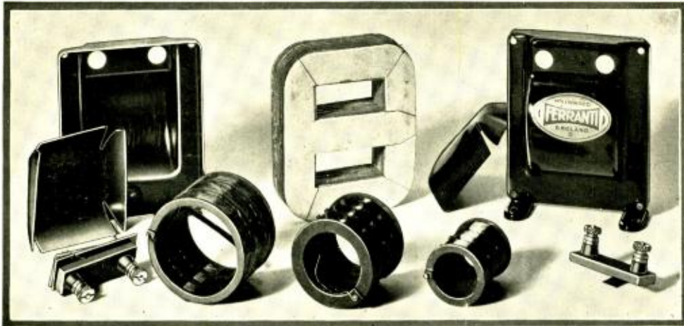
Components of Ferranti Transformer
