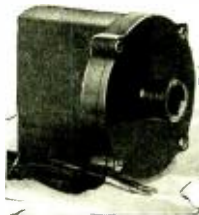
B. A. 1. Balanced Armature Unit 3 11/16" x 3 5/16".
