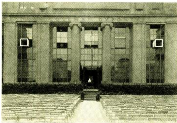
Fig. 4. A typical public address projector installation. Two large speakers can be seen protruding from the end windows in the building.
