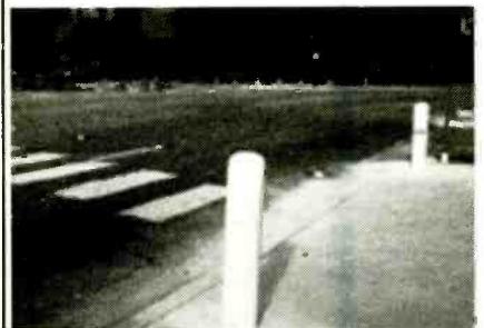
To activate the system in a typical setup, pedestrians simply walk between two Bollards at the top of the crosswalk.
