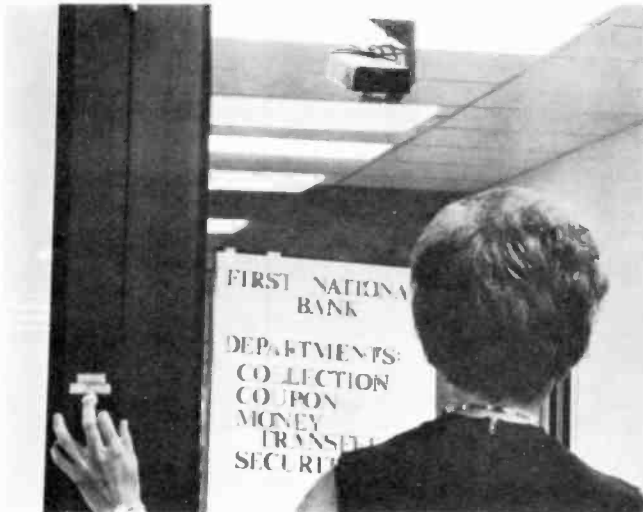
BANK EMPLOYEE pushes button at door for admittance. CCTV camera and intercom provide visual and voice identification to guard who monitors activities in building and controls the door.
