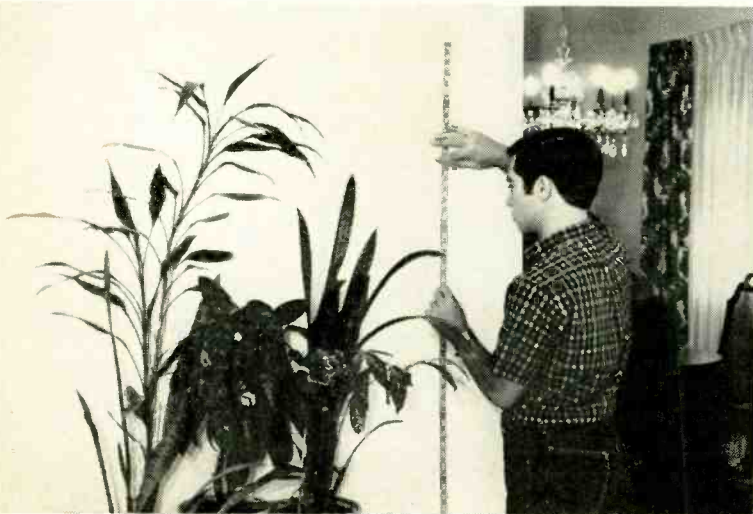
Fig. 4—Mark off the area to be cut out as accurately as possible. Do not depend upon the panel escutcheons to hide sloppy work.
