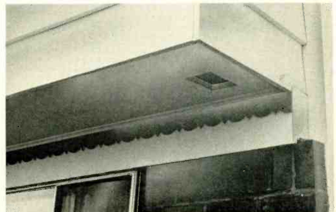
Fig. 9—More than adequate gain and sensitivity permitted locating the front door unit under the overhang, away from rain.
