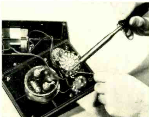
Construction of Multimeter.
