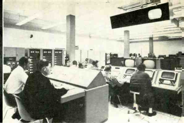
Control room at the Andover ground stations keeps careful track of operation. Consoles (foreground) track Telstar. Monitors (right) evaluate signal levels during transmit and receive tests to satellite.
