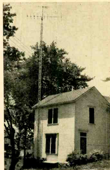
Fig. 3—A 54-foot steel tower installed near two-story house.
