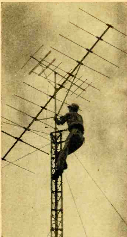
Fig 6—Using safety belt on tower.
