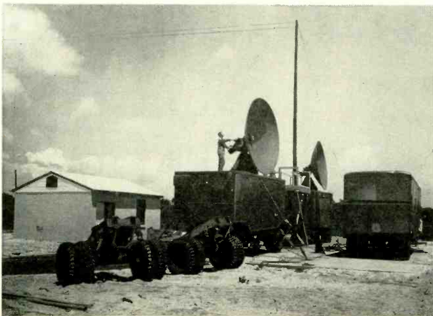
Air Force mobile radar installation.
