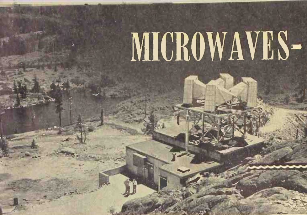
Fig. 1. The Cicco-Brite, Calif. station of the transcontinental microwave relay system installed by AT&T for transcontinental telephone and television service.
