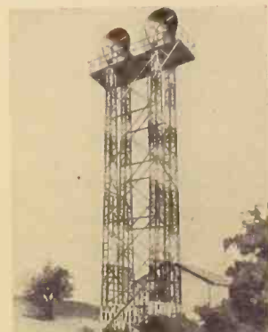
One of towers used in first commercial microwave telephone circuit, between England and France, opened in 1933.
