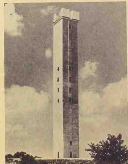
A concrete microwave relay tower. Lens antennas are used in this system.
