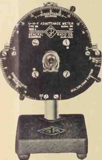
The u.h.f. admittance meter for direct reading of admittance and susceptance.
