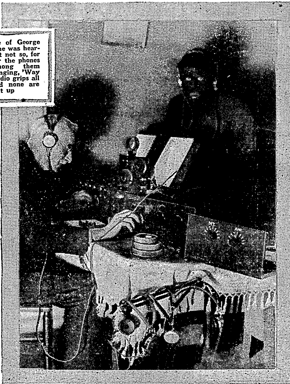
Little Miss Wagoner listens in on a new Radio receiving set which is operated with the new peanut tube. The set is entirely void of storage cells © Int.
