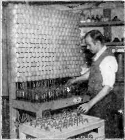
Fig. 3: An "ageing rack" used in the experimental tube laboratory. Here different tubes are subjected to different loads and their behavior observed.
