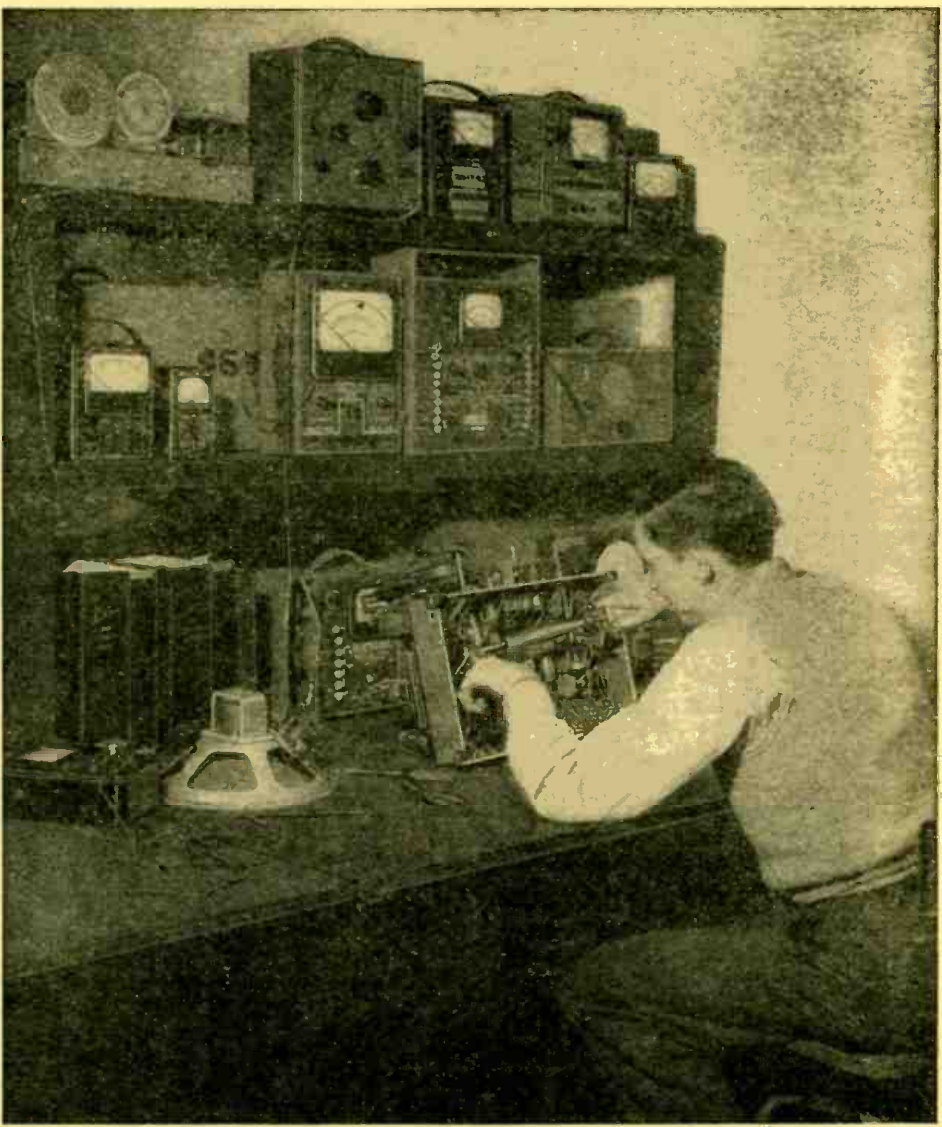
Work on the new Sams' test bench. Left portion is part of a second identical bench used to double length. The large stock of meters represents part of Sams' equipment-testing program.
