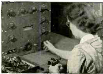
Every carbon element that goes into Mallory controls is individually inspected to be sure that its resistance value is the same as specified on the labels.
