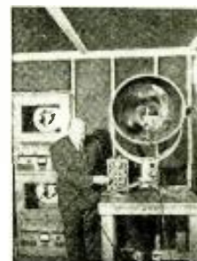
Allen B. DuMont and the Photovision transmitter. Upper picture is relayed by Photovision, lower is direct from transmitter.
