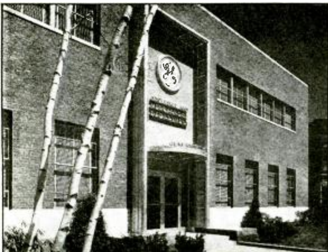
Visitors to General Electric in Bridgeport must enter this door & pass through a reception lounge & display of appliances in order to reach factory & offices beyond. Building also houses testing lab & meeting room.
