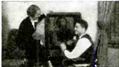
Repairing Radio Sets
