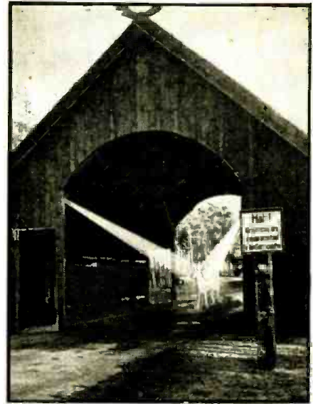
Fig. A. The animal in the above photo has just interrupted the light beam and is startled by the sudden glare of 2 floodlights and the blaring of an automobile-type horn! In a flash he will be scared back into the preserve ground.
