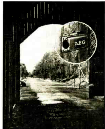
Fig. B. This is an interior view of one of the arches looking toward the preserve grounds. Notice how the exciter-lamp housing is placed to throw the beam of light across the entrance. The insert is a close-up view of the exciter lamp housing. Motor vehicles do not actuate this "robot guard"; only animals "touch it off."
