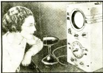
Singer testing pitch of her voice by observing waveform on cathode-ray screen of resonoscope.
