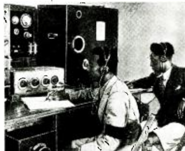
The Ethiopian radio station installed at Harrar.
