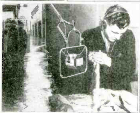
In the studios of Germany's new Koenigsberg station are employed extensive means to secure a low angle of incidence, in order to obtain an optimum echo time. Ceilings are equipped with tilted areas of planking that prevent direct reflection; similarly, the walls are built as sections, slanting in a horizontal plane. Globe Photo
