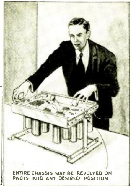
This rack, for rotating and supporting radio chassis, is excellent for Service Men.
