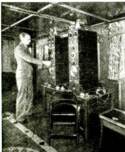
Left—The two short wave transmitters for sending press reports on the race. Below—The sequence of incidents in locating a man by amateur radio.
