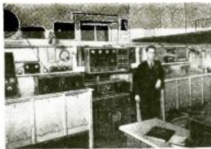
Servicing equipment on a "trolley line."
