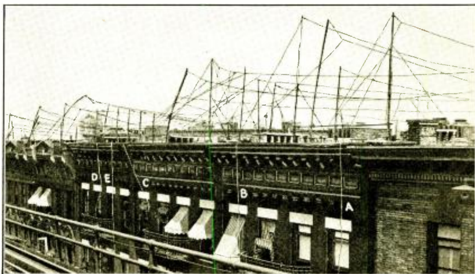
Fig. A A typical sky-line of New York. Lead-ins A, B, C, and D run directly in front of the windows, not only marring the appearance of the buildings but actually causing a fire hazard where they run in front of fire escapes.
