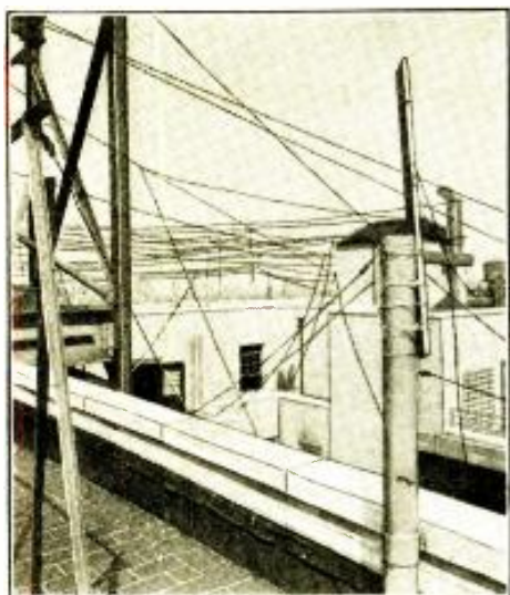
Fig. B The pipe which caused a "shower of plaster."
