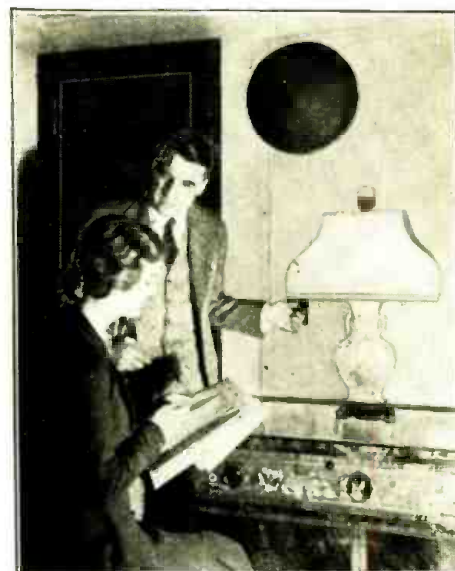
A typical room installation in the New Yorker Hotel. The wall plate under the man's hand contains the four-station selector switch and volume control; the reproducer cone is above it.
