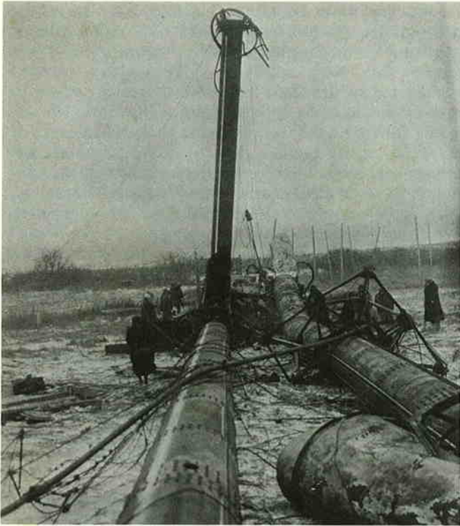
The 420-foot mast of station BO at Brant Rock, Mass., photographed immediately after it was deliberately toppled by order of the U.S. Navy in December, 1917.
