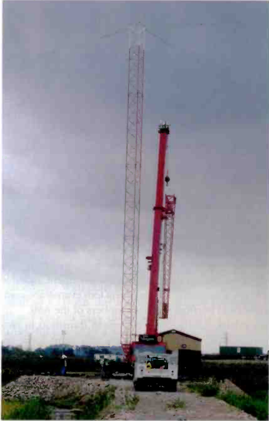
The first 100' of tower going up
