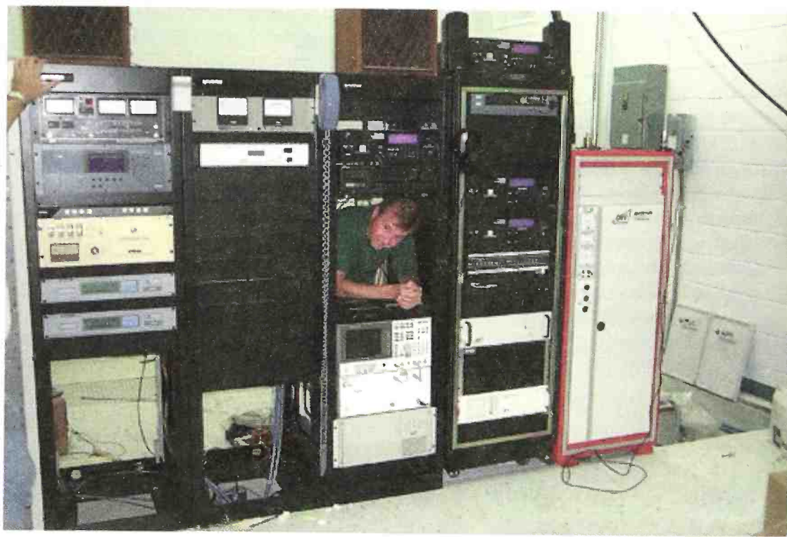
Walden strikes a pose behind the FM IBOC installation at WMMO in Orlando before the radio show.
