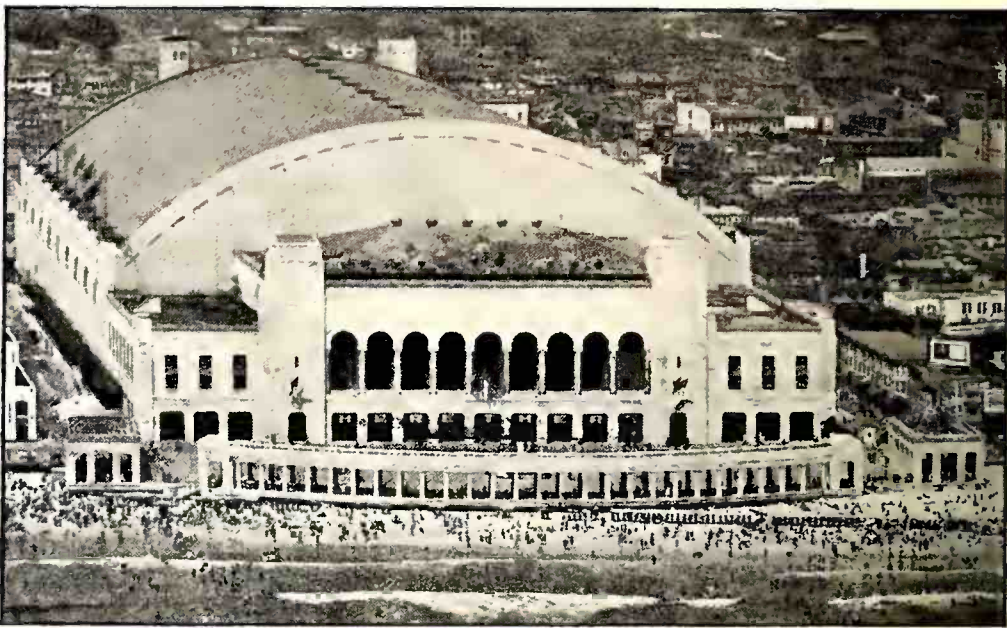
The new mammoth $15,000,000 civic auditorium on the boardwalk at Atlantic City where the Annual Convention and Trade Show of the Radio Manufacturers' Association will be held during the week of June 2. The building is the last word in convention hall construction. It is 350 feet wide by 650 feet deep and provides 85,000 sq. ft. of exhibition space.
