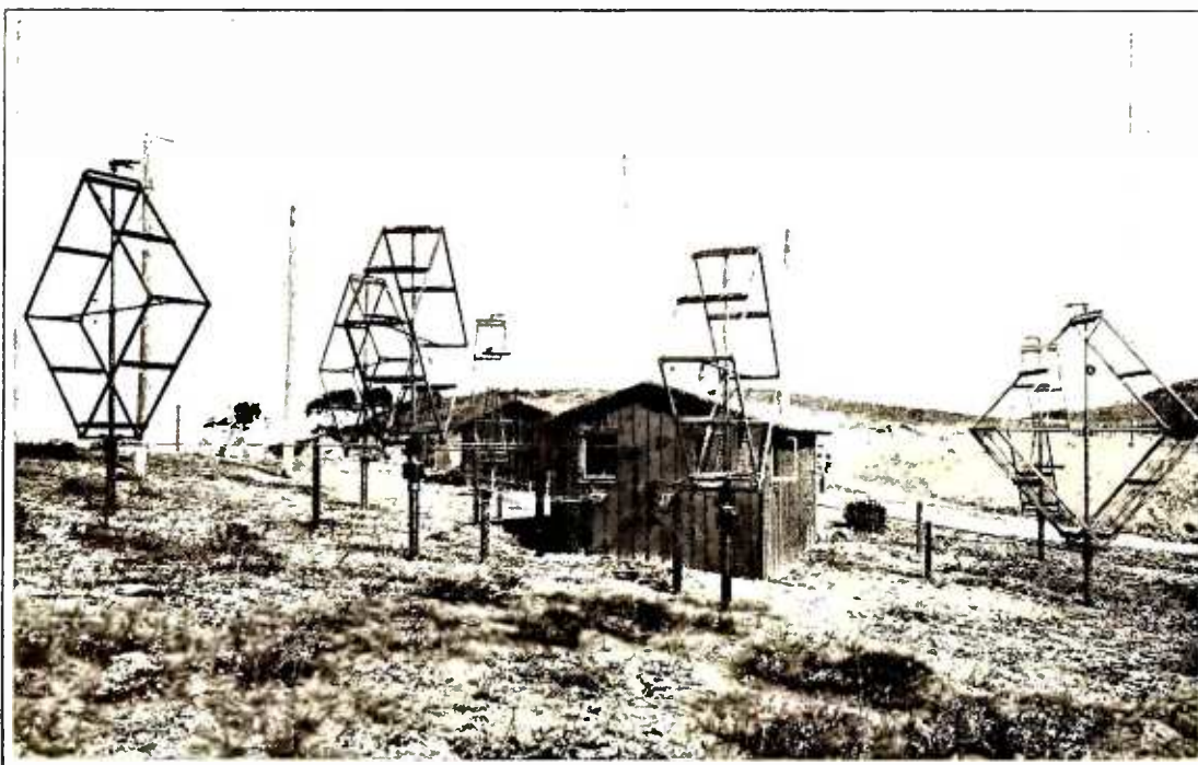
VIEW OF SAN FRANCISCO RECEIVING STATION AT DALY CITY, CALIFORNIA, SHOWING ROTABLE LOOP AERIALS. THIS STATION IS OPERATED BY THE FEDERAL TELEGRAPH FOR THE RECEPTION OF MARINE SIGNALS
