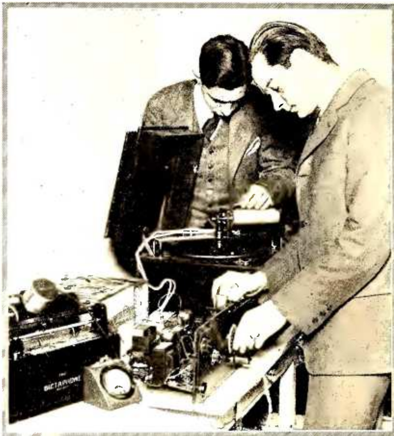
The author receiving pictures by means of a Cooley Rayfoto receiver
